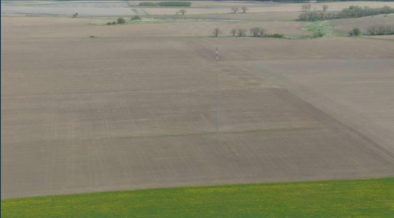
MET towers or Meteorological towers are used to gather wind data necessary for site evaluation and development of wind turbine projects. They can be erected very rapidly and may be on site from a few days to up to a year or longer. At this time there is no standardized notification system in place to indicate when and where these towers are erected.
