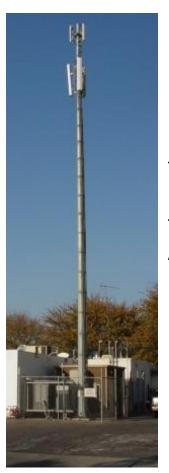
Monopole Tower- A monopole tower is a single tube tower. It requires one foundation and typically does not exceed 200' AGL.
