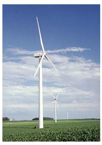
Wind Turbines – large 1.5 to 3.5MW wind turbines typically used in this area are 200' to 300' AGL with blades reaching another 120 to 150'. Usually arrayed in wind farms.
