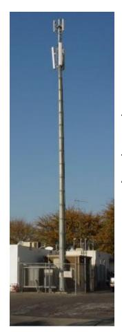
Monopole Tower- A monopole tower is a single tube tower. It requires one foundation and typically does not exceed 200' AGL.
